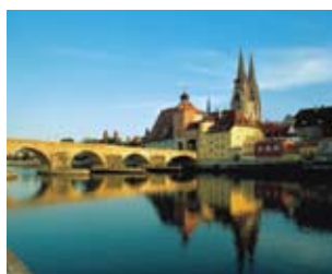
Regensburg Stone Bridge
